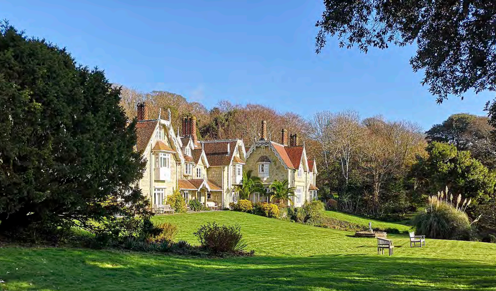
Figure 7.7: Captain Pelham's Cottage, now Lisle Combe (November 2019). [Kate Feluś]
