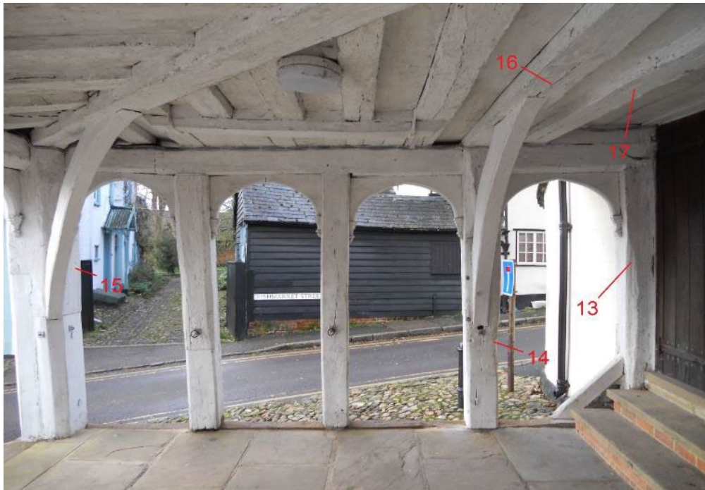
Figure 9: Photograph looking west showing some of the timbers sampled from the covered market area (photograph Martin Bridge)
