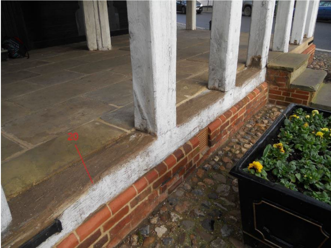
Figure 11: Photograph of the front left side of the covered market area, showing the sill plate sampled for dendrochronology (txgh20) (photograph Martin Bridge)
