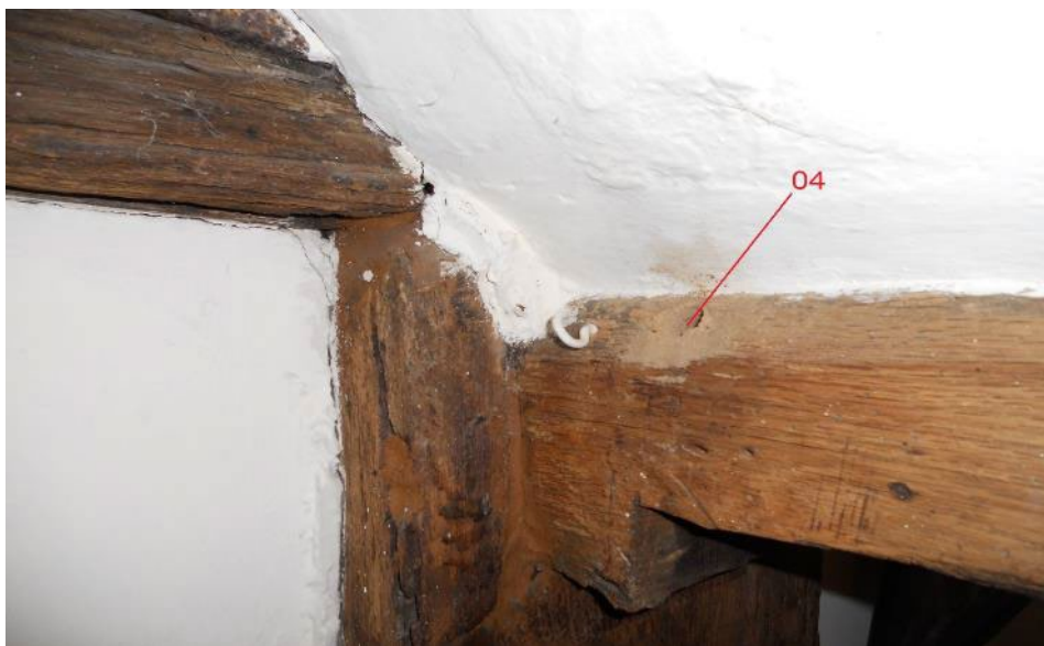
Figure 4: Photograph of the south (front) end of the central valley wallplate showing the position of coring through complete sapwood (photograph Martin Bridge)
