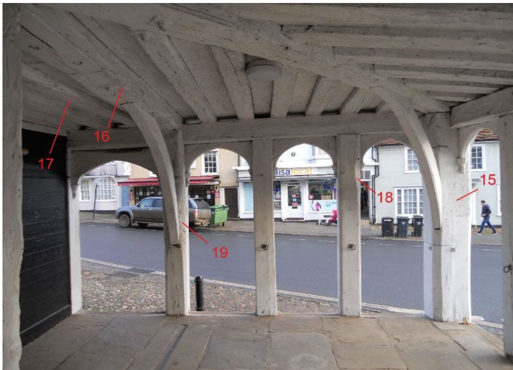
Figure 10: Photograph of the right-hand side of the covered market area showing timbers sampled for dendrochronology (photograph Martin Bridge)
