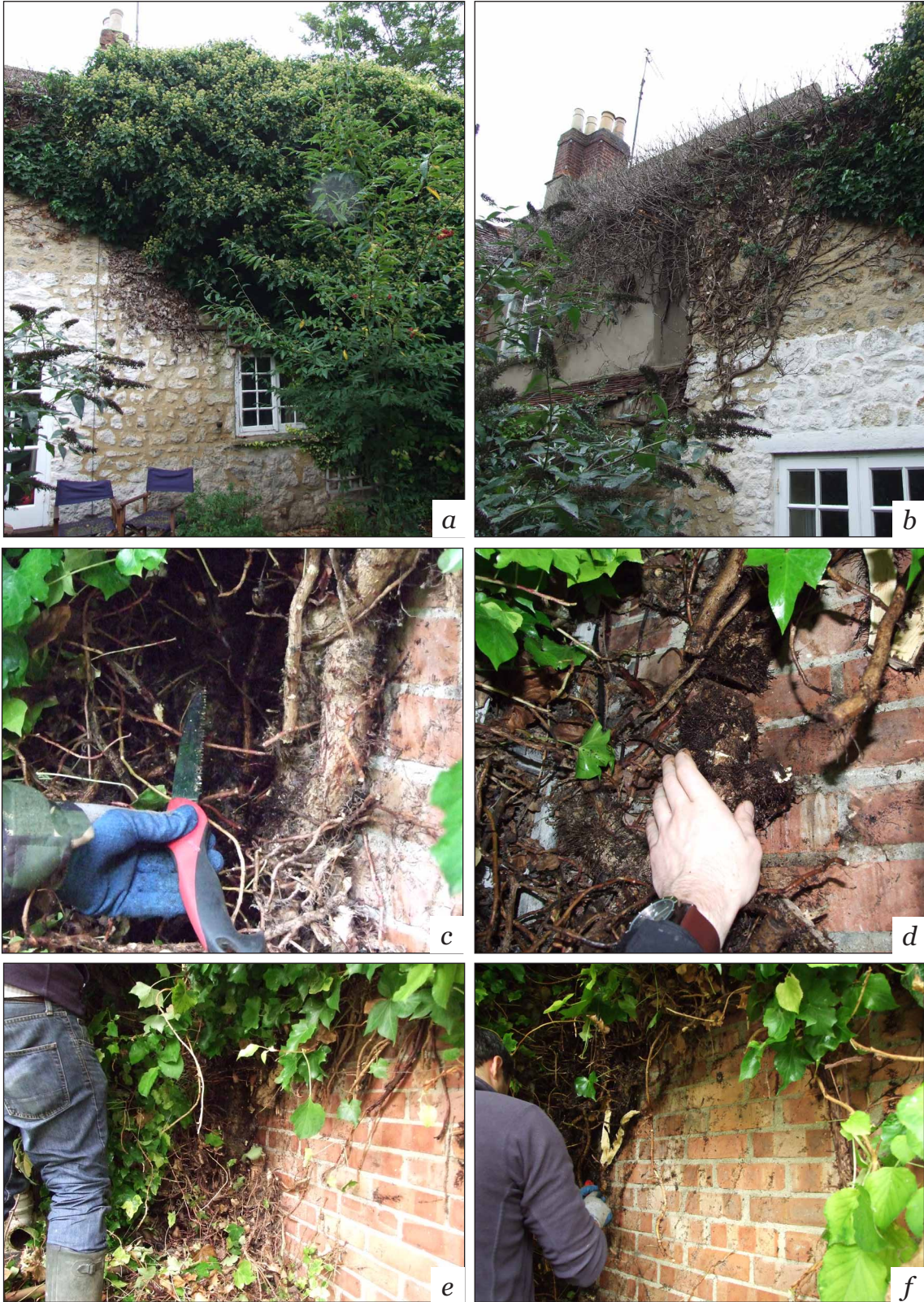
Figure 4-1. Photographs of ivy and its management on a stone and brick cottage, Walton Street, Oxford.
