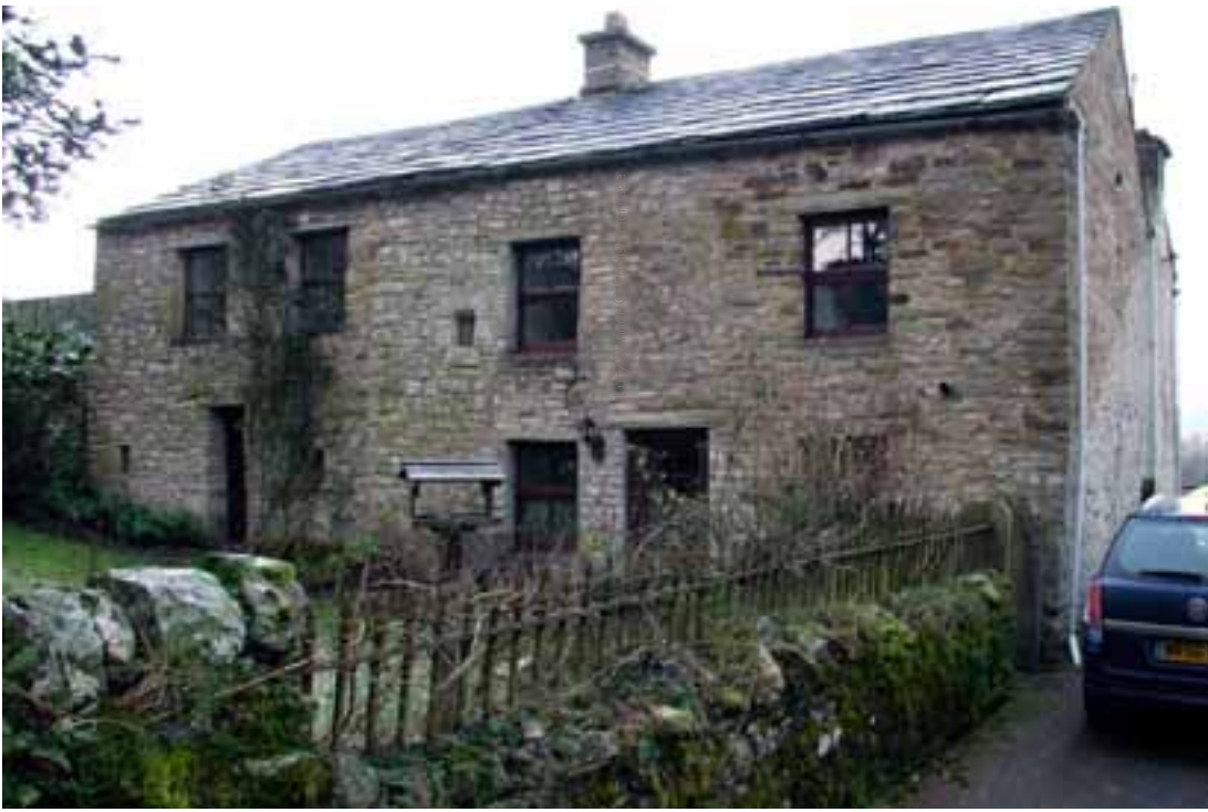
Nettle Hall, Galligill: the 17th-century house-over-byre with its chamfered first-floor fire window surround has been extended to the left in the 18th century and to the rear in the 19th century, at which point it was totally re fenestrated and much of the front wall was rebuilt
