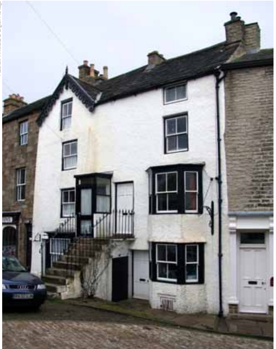
Above: Cross View, Market Place, Alston. This pair of houses hide an interesting history behind their later 19th-century elevations. That to the left retains its late 17th-century walling facing the churchyard, with traces of chamfered window surrounds. As rebuilt, they retain the local distinction between principal living accommodation on the upper floor, reached by an external stair, and a separately-entered ground floor, which appears to have been in domestic occupation and is currently used as a shop
