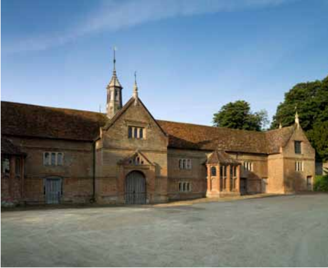
The north front of the stable building at Audley End
