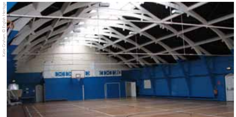
The interior of the Drill Hall, showing laminated trusses
