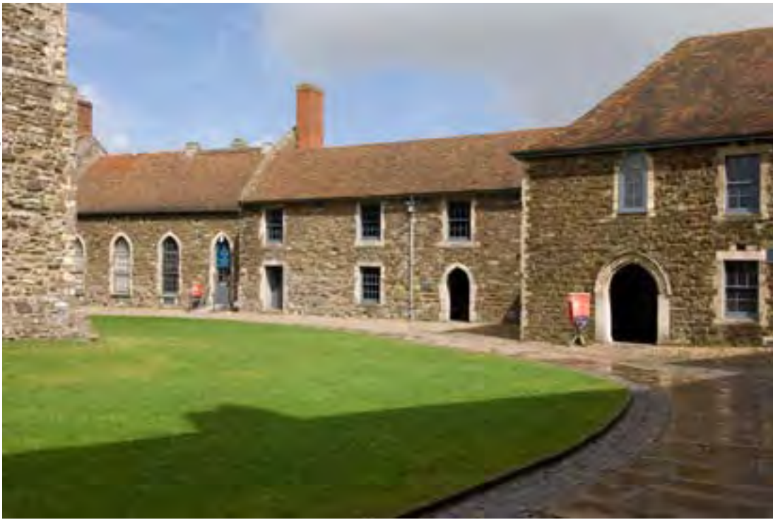
Buildings of north-east side of Inner Bailey - Arthur's Hall in centre
