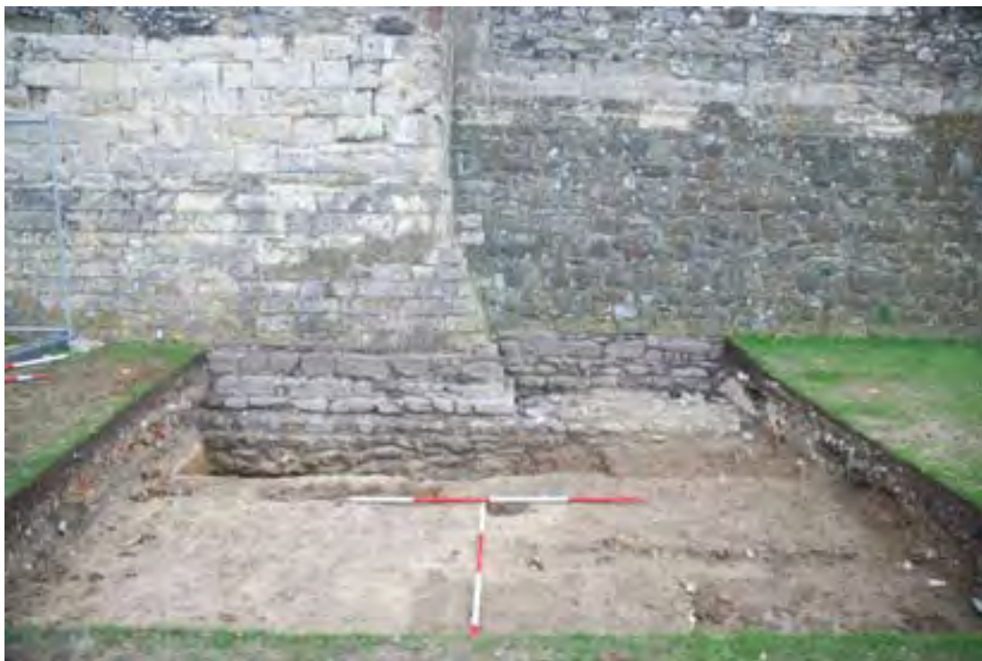
Trench A showing Great Tower footings, Caen-stone surface (foreground), and sondage against wall to expose early construction evidence
