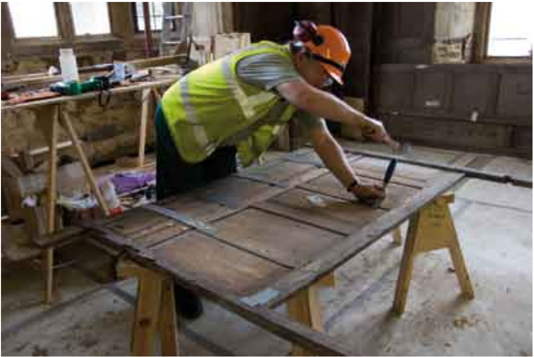
Martin Stapleton repairs the wooden panelling from the Long Gallery
