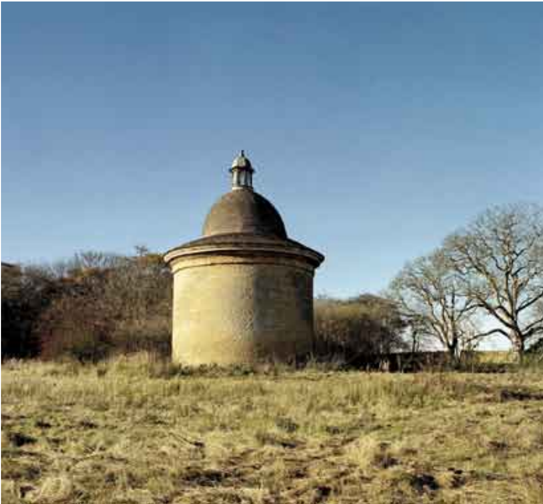
The Dovecote. One of the most significant features of the designed landscape is the Dovecote, built in 1739/40 on rising ground 200m to the north-west of the Hall, and part of the 7th Earl's embellishment of the estate. The Dovecote, with its distinctive ogee roof profile, was designed as an eye-catcher or feature in the park and is visible across much of the southern and eastern areas of the garden
