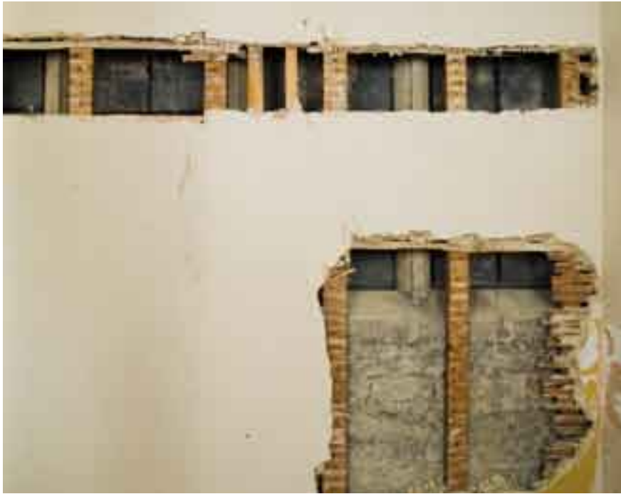
This partially uncovered window lit the Great Chamber in the 1560s, and was blocked in the 1740s
