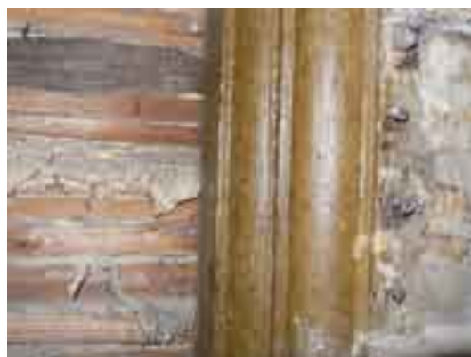
Wooden architrave of Duke's Chamber
