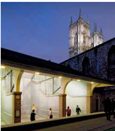
8.4 Westminister School, Eton fives courts © English Heritage Archive
