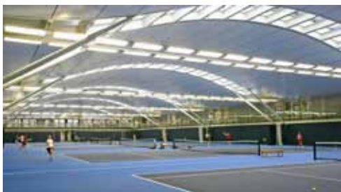
33.28 Interior of National Tennis Centre © Lawn Tennis Association
