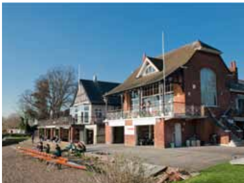
19.4 University of Westminster boathouse (right) with Ibis boathouse (19.3) on left © English Heritage Archive
