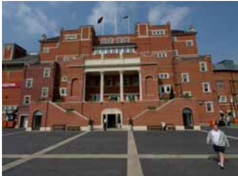
23.1 Oval pavilion exterior, following its refurbishment in 2013
