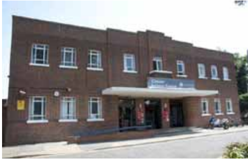
30.11 Cheam Leisure Centre entrance before refurbishment in 2014 © LB of Sutton
