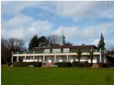
25.11 former Oberon Athletic Pavilion, Lindisfarne Road, now Hall School © Simon Inglis / Played in Britain
