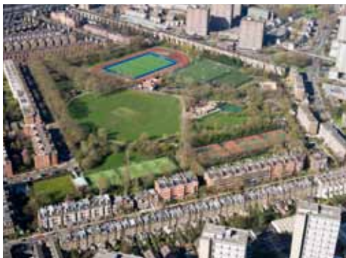
8.14 Paddington Recreation Ground © English Heritage Archive
