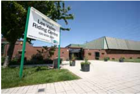
32.7 Lee Valley Riding Centre exterior © Andy Howe / Lee Valley Regional Park Authority
