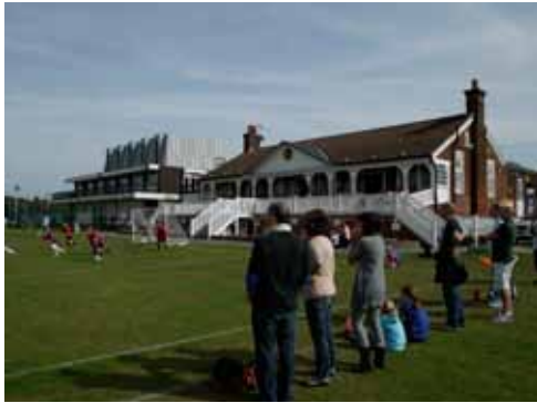
5.5 Pavilion at Goals Soccer Centre, former Three Banks sports pavilion
