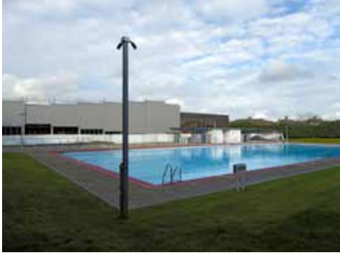
15.7 Park Road open air pool with indoor pool and leisure centre in mid-reconstruction in background
