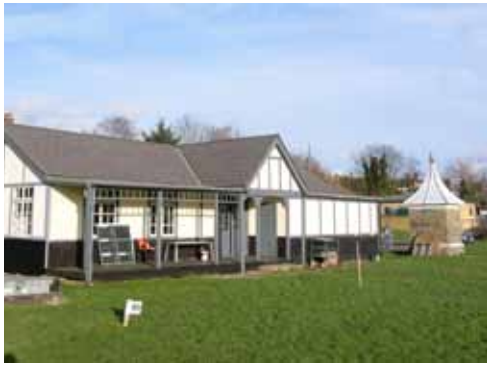
15.5 former pavilion at Aquarius Archery Club, before it was destroyed in arson attack, 2012. To the right is a square brick building (c.1908) providing access for testing the reservoir below © Simon Inglis / Played in Britain
