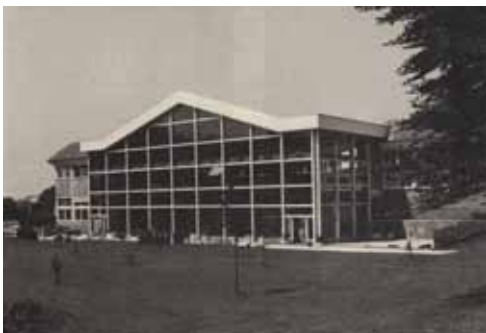
33.15 Bank of England Sports Hall and Swimming Pool after its completion in 1970 © Bank of England Sports Club
