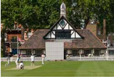
8.3 Westminister School pavilion, Vincent Square © English Heritage Archive
