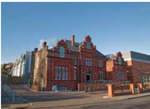
24.2 Former Ladywell Swimming Baths with new leisure centre to right and new pool to left at rear. © Simon Inglis / Played in Britain
