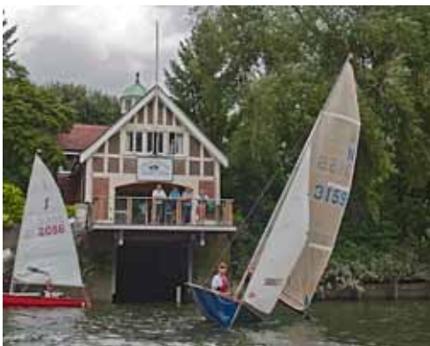
28.4 Twickenham Yacht Club, showing mezzanine and balcony inserted within original arched docking area © Simon Inglis / Played in Britain
