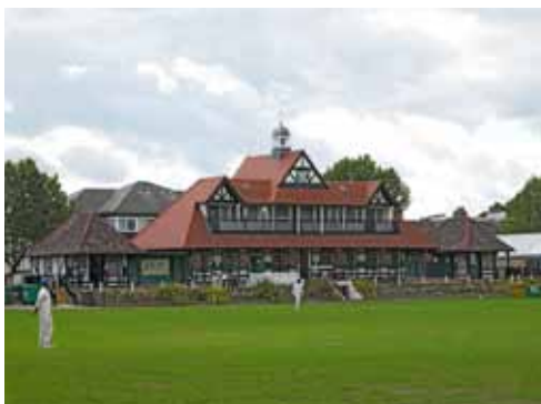
32.2 Pavilion at Leyton County Cricket Ground © Simon Inglis / Played in Britain
