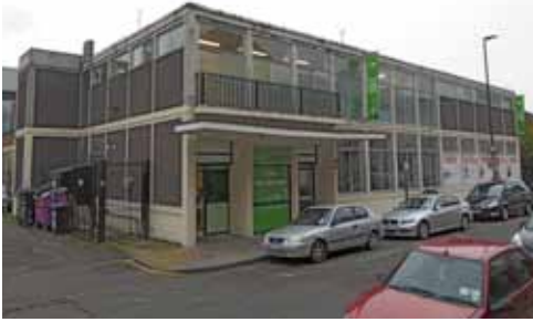
31.3 Tiller Leisure Centre exterior
