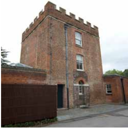
28.1 Tiltyard Tower at Hampton Court Palace © Historic Royal Palaces
