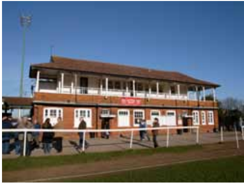
28.11 South elevation of pavilion at Richmond Athletic Ground © Simon Inglis / Played in Britain
