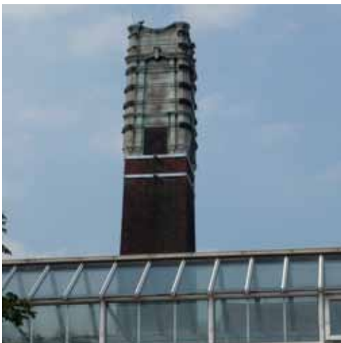
10.2 Acton Baths chimney (before construction of new sports centre on site) © Simon Inglis / Played in Britain
