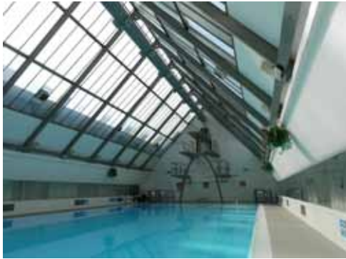
29.9 Swimming pool at former Pioneer Health Centre, now Frobisher Place flats
