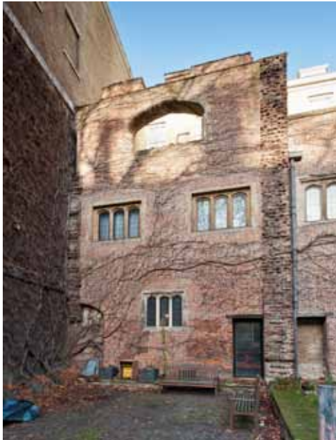
8.1 Surviving northern wall of tennis court at Whitehall Palace, now part of Cabinet Office, Treasury Green, Downing Street
