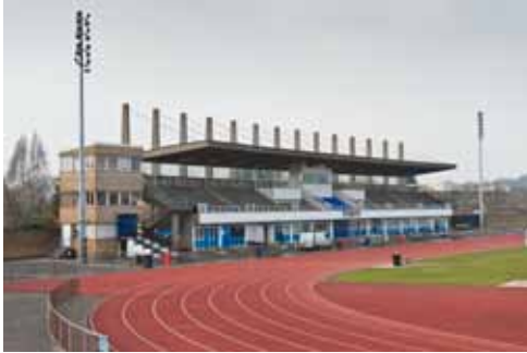
2.3 Copthall Stadium / Allianz Park grandstand © English Heritage Archive
