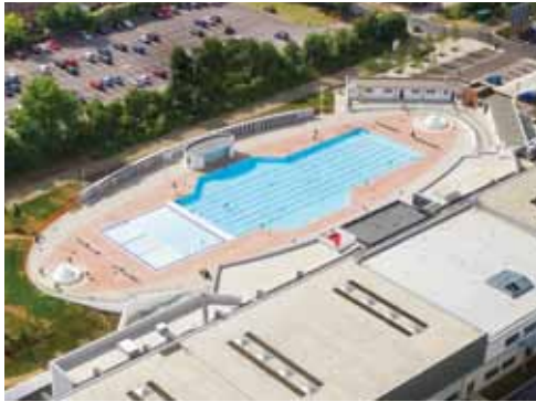
18.3 Hillingdon Outdoor Pool, with children's pool on left, indoor facility in foreground and entrance block top right © Flag-Soprema UK
