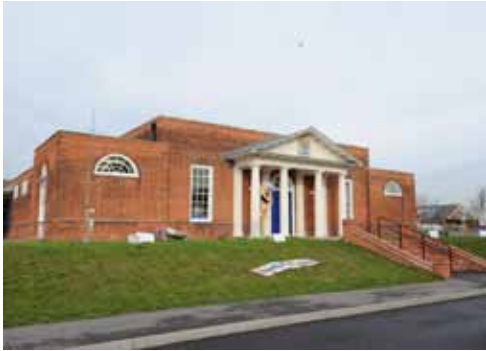
27.1 Former sports pavilion of the Port of London Authority, now Cranbrook Lane Primary School © Simon Gill / Played in Britain
