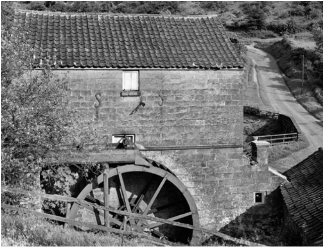
Figure 5 An unidentified mill with an overshoot waterwheel. Water ran onto the top of the wheel which rotated clockwise.
