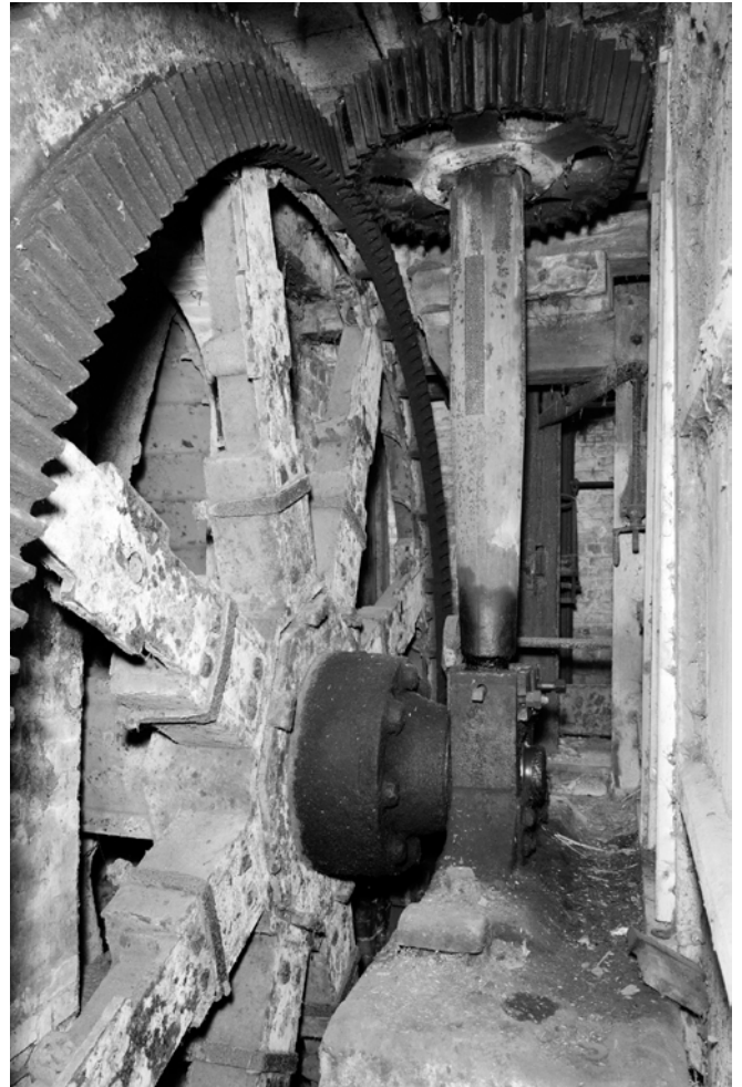
Figure 7 Early modern mill gearing, Narborough Mill, Norfolk. The waterwheel can be seen through the large vertical gear which it turned directly. The rotation was then transferred through 90° by the small gear and a shaft ran up to the room above to turn a millstone.
