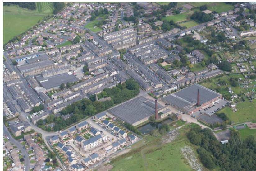
The industrial settlement of Harle Syke near Burnley, provides a fine example of an historic industrial townscape of the Lancashire weaving district © Historic England
