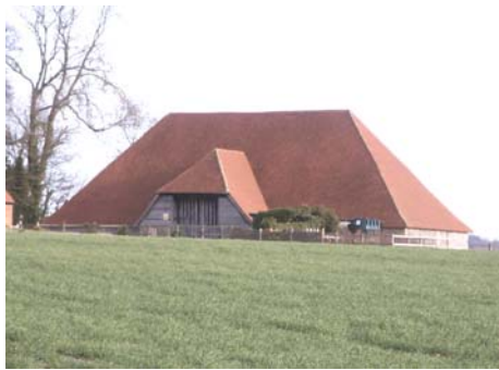
Aisled Threshing barn demonstrating the dominance of the roof over the walling
