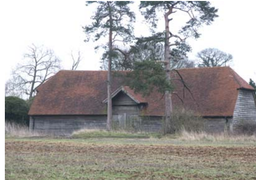
Five bay timber-framed aisled threshing barn typical of many barns found in the Character Area.
