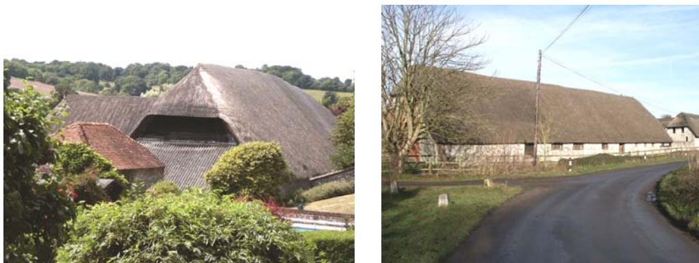
Long straw thatch with flush ridges and sparred eaves on two large threshing barns that are characteristic of the Hampshire Downs
