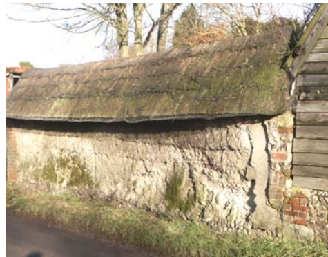
Cob boundary wall with thatch capping
