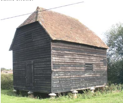
Timber-framed two-storey granary
