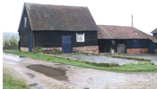
Timber-framed and brick stable
