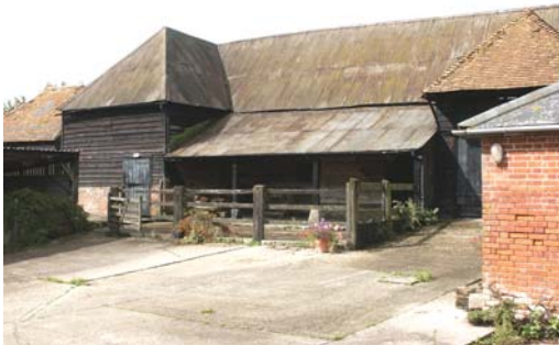
Timber-framed threshing barn with lean-to cattle shelter
