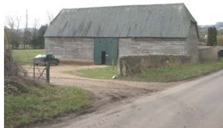
19 th century unaisled threshing barn
