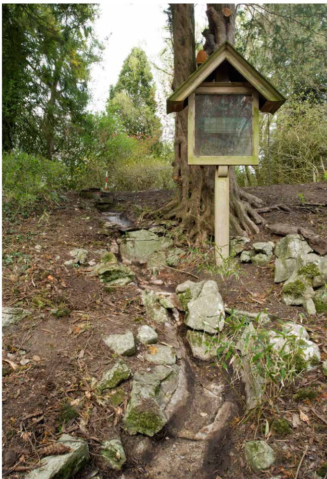
The narrow concrete waterfall channel, now dry. © Historic England, Alun Bull
