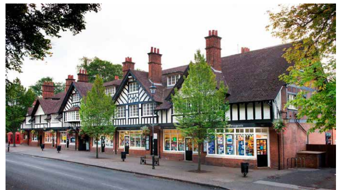
37-47 Sycamore Road, Bournville, West Midlands, built in 1905-8 to designs by E Bedford Tyler and listed Grade II. © Historic England, James O Davies
