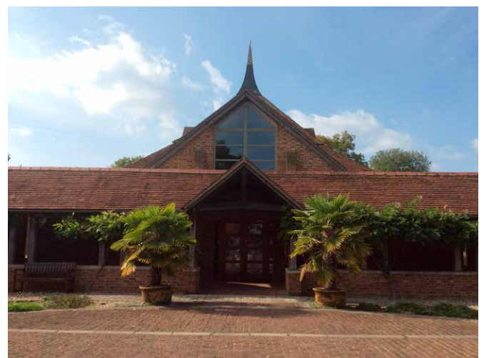
The library at the Amaravati Buddhist Monastery, Hertfordshire. The earliest buildings here were constructed as part of a children's camp in the 1930s.
