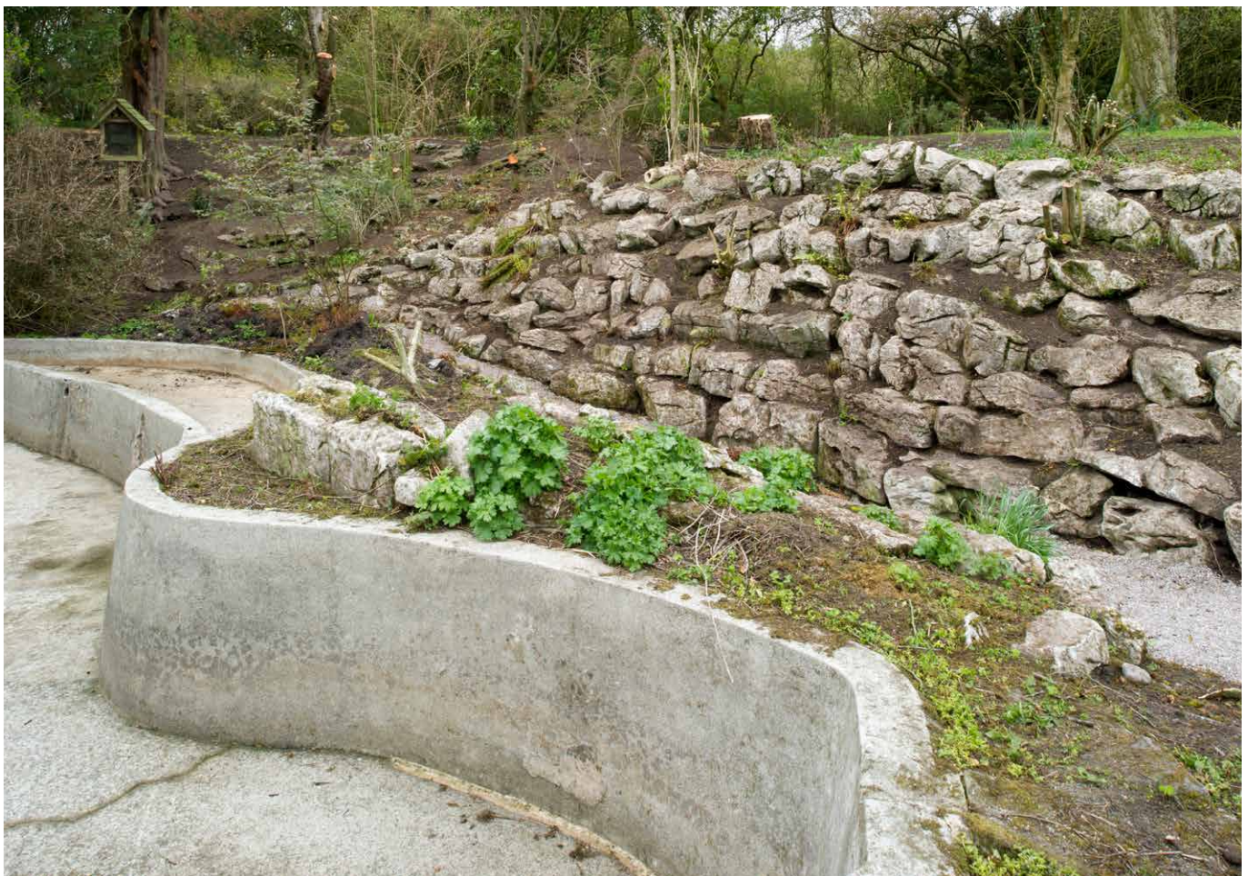
The pond with concrete bog garden shelf and rock face beyond. © Historic England, Alun Bull
