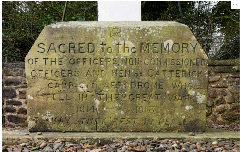
Figure 13: Memorial near Catterick, North Yorkshire. Legibility is impaired by the heavy algal growth.
