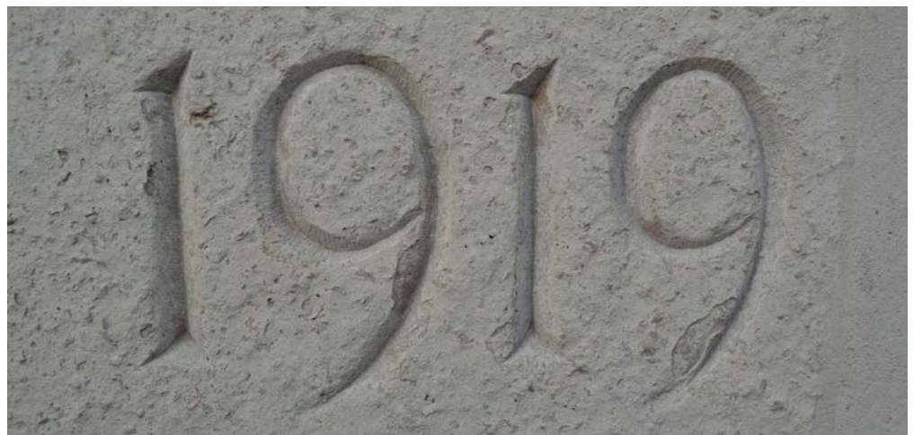
Figure 4: Stockwell war memorial, Lambeth Road, London. Incised lettering in Portland stone. The marks of the chisel are evident on each side of the 'V' cut of the letters.
