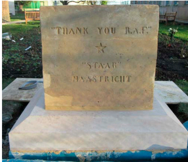
Figure 23: Biggin Hill Memorial Museum, Biggin Hill, London. A thin sheltercoat applied to a war memorial made of Maastricht limestone provides a sacrificial, breathable and protective coating to the stone.
