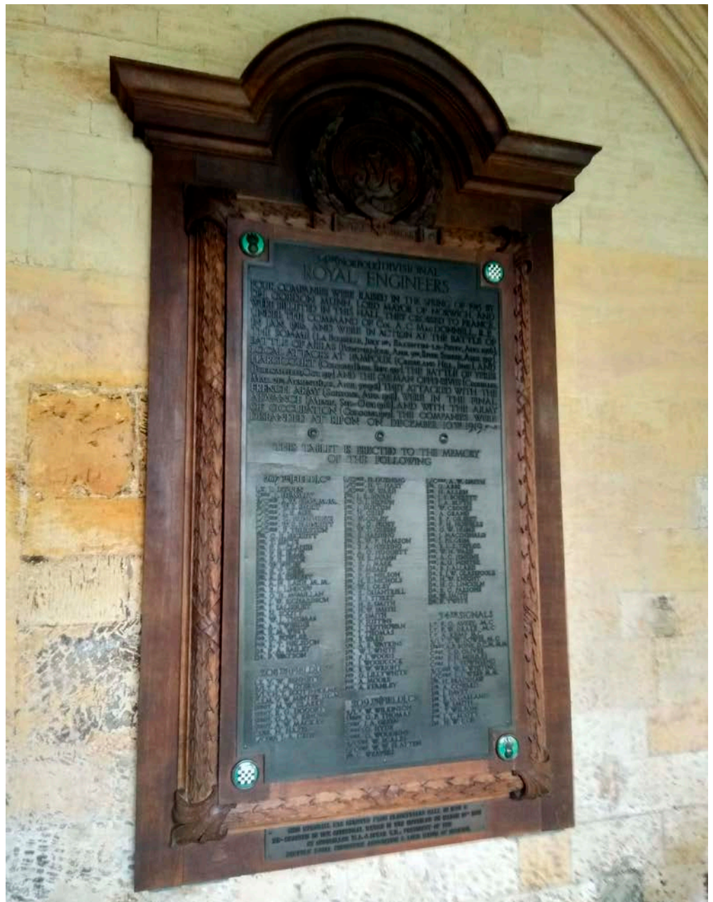
Figure 34: Norwich Cathedral cloisters, Norwich, Norfolk. The badges in the lower two corners have been cast in resin from moulds taken from the bronze ones at the top.
