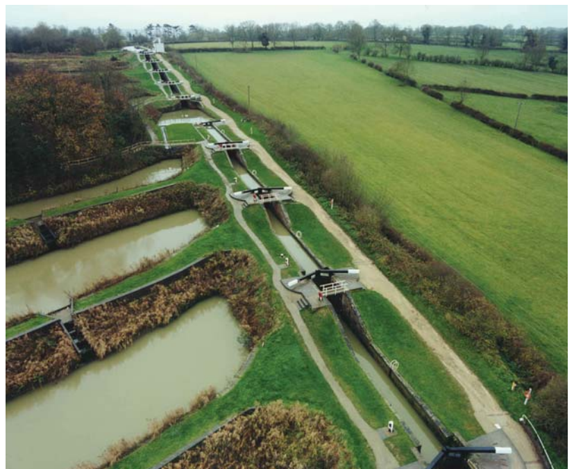
The Foxton flight of locks in rural Leicestershire. This important structure is designated as a conservation area and a management agreement has recently been developed for the site. © British Waterways
