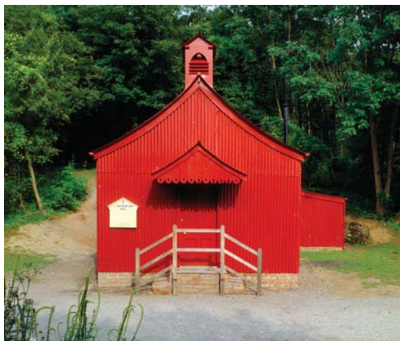
St Chad's Mission Church, Madeley, Shropshire, an example of a prefabricated building of corrugated iron. Photographed by Eric de Maré between 1978 and 1980 and now accessible through the ViewFinder website. © English Heritage.NMR
