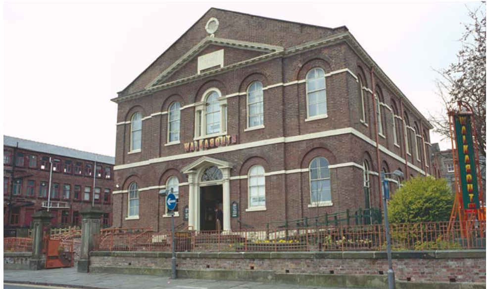
The former Wesleyan chapel, Carver Street, Sheffield. The chapel was built in 1804–5 to designs by the Revd William Jenkins, and was recently sold for conversion into a pub. © Mrs Barbara A West LRPS (Images of England 456194)
