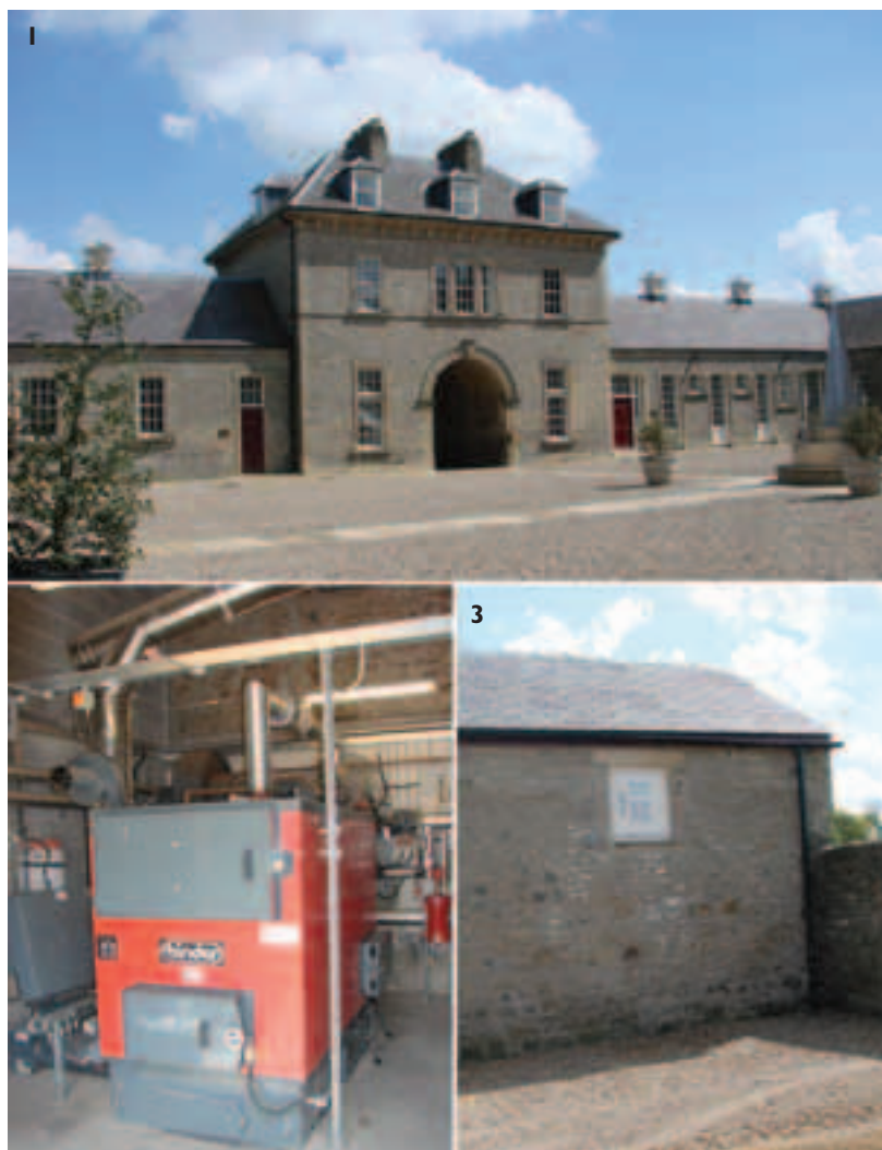
At Aske Hall, near Richmond in North Yorkshire, wood-chip boilers are being progressively installed as more efficient and environmentally friendly replacements for traditional heating systems. 1: Aske Hall stableyard, 2: wood-chip boiler, 3: traditional building used as a hopper for the wood chip. © Historic Houses Association
