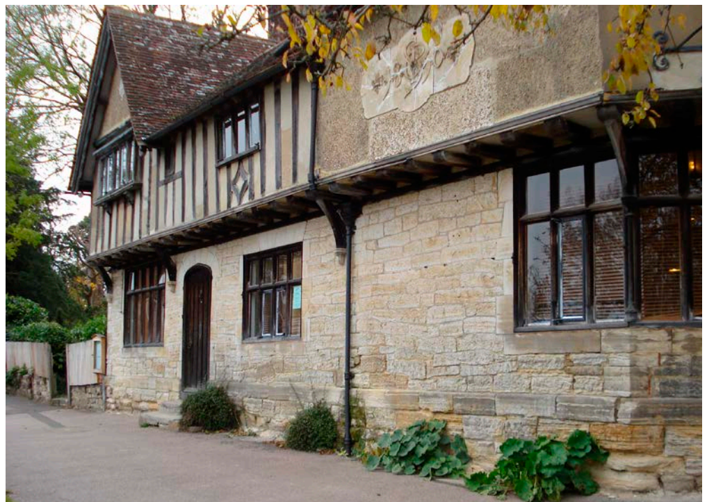
Figure 3: Timber frame and stone building, Penshurst. Wealden Group Sandstone.
