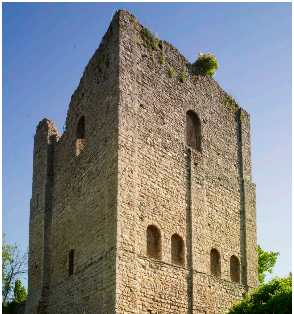
Figure 25: St Leonard's Tower, West Malling. Tufa quoins and dressings.
