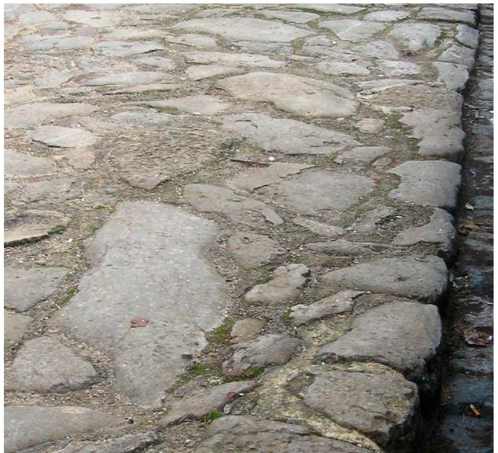
Figure 8: Paving, kerbing and channel blocks, Biddenden. Wealden Limestone.
