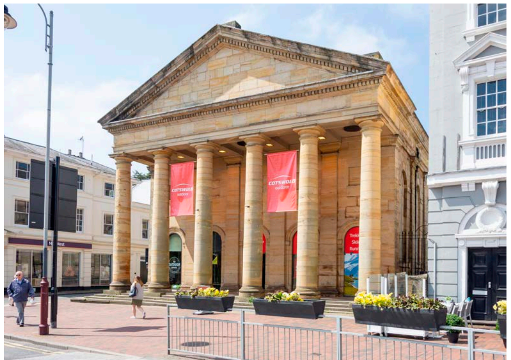
Figure 2: Lecture Hall, Tunbridge Wells. Wealden Group Sandstone.
