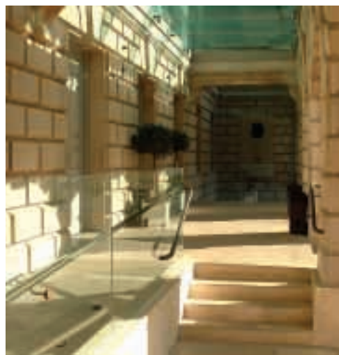
New access ramps at the Royal Academy of Arts
