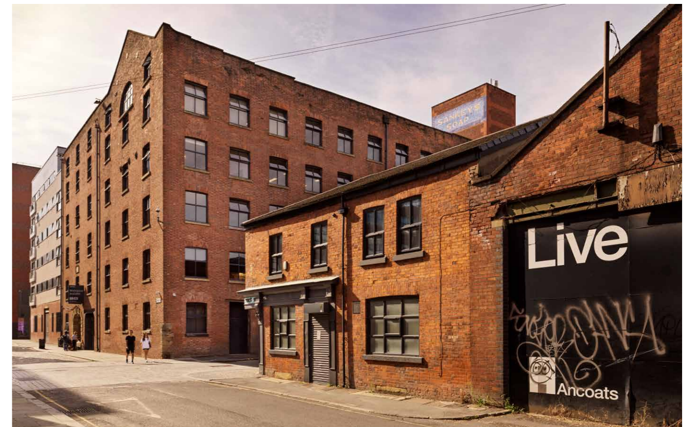
Beehive Mill, Jersey Street, Ancoates, Manchester, Greater Manchester. © Historic England Archive
