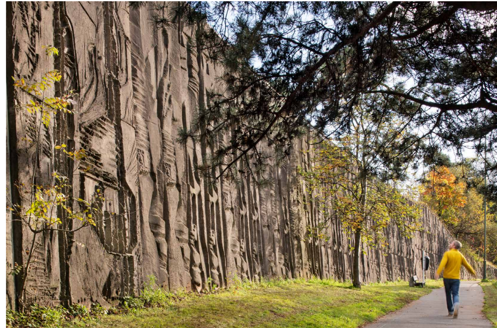
The prolific architectural sculptor William Mitchell designed this decorative retaining wall by the Kidderminster inner ring road. © Historic England Archive
