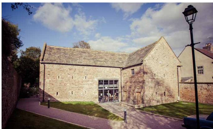
Dronfield Hall Barn. © Red Snapper Photography
