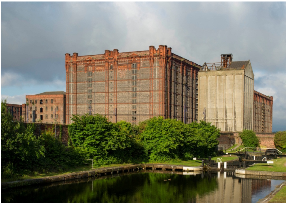
Work begins on the Tobacco Warehouse at Stanley Dock, Liverpool. © Historic England
