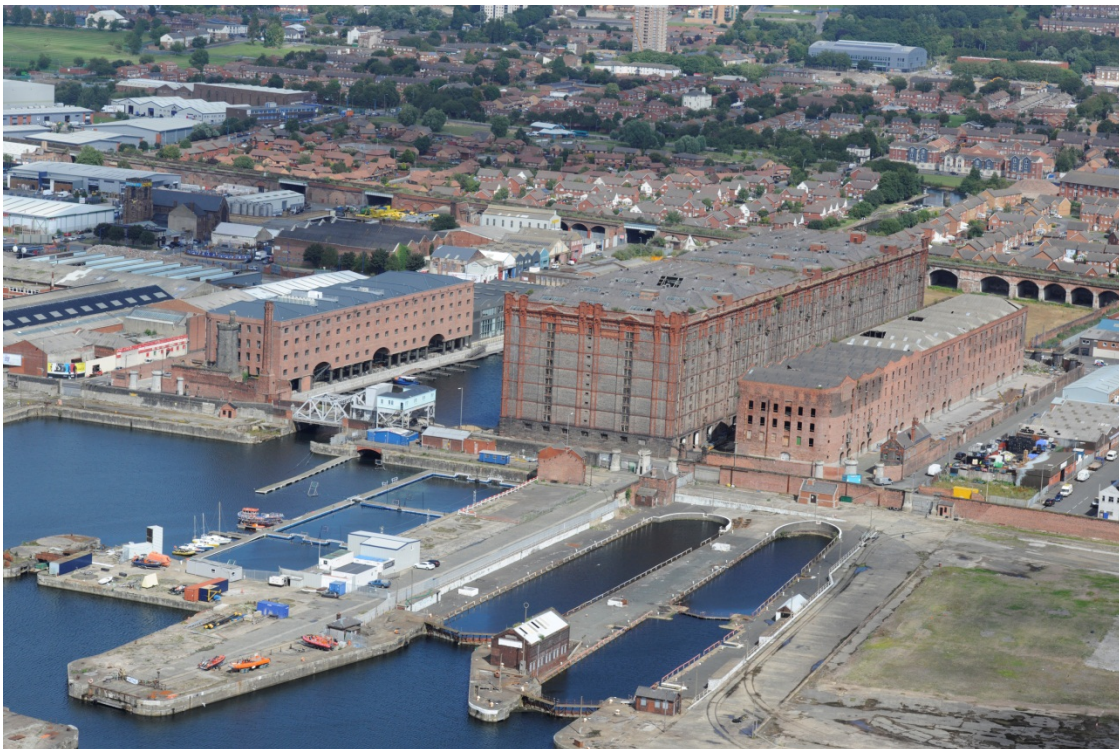
Aerial view of the three main warehouses at Stanley Dock in Liverpool. © Historic England
