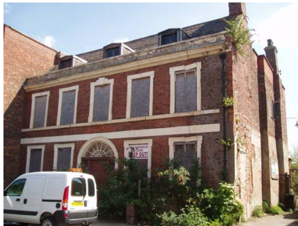
116 High Street, Boston before regeneration 2009 © Heritage Trust of Lincolnshire and Gleeds
