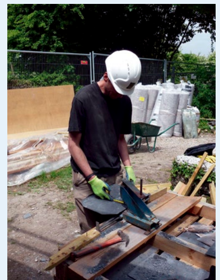
Trainee Rob cutting slate at Heron Corn Mill, © Alan Gardner Associates
