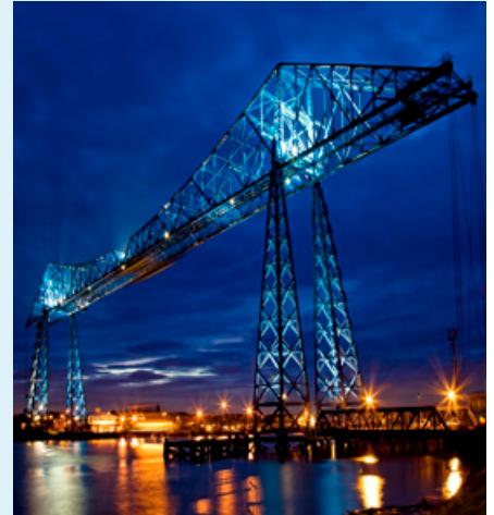
Middlesbrough Transporter Bridge © English Heritage
