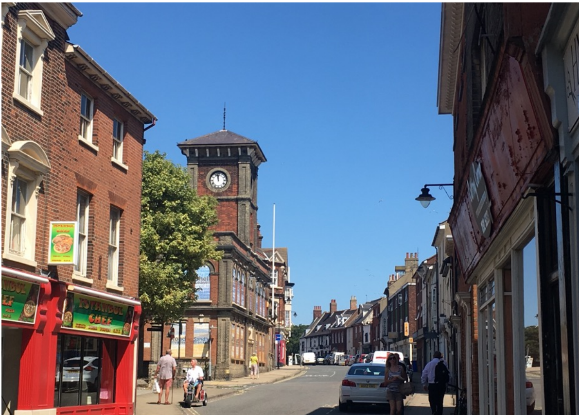
Figure 9: Town Hall from the High Street looking north
