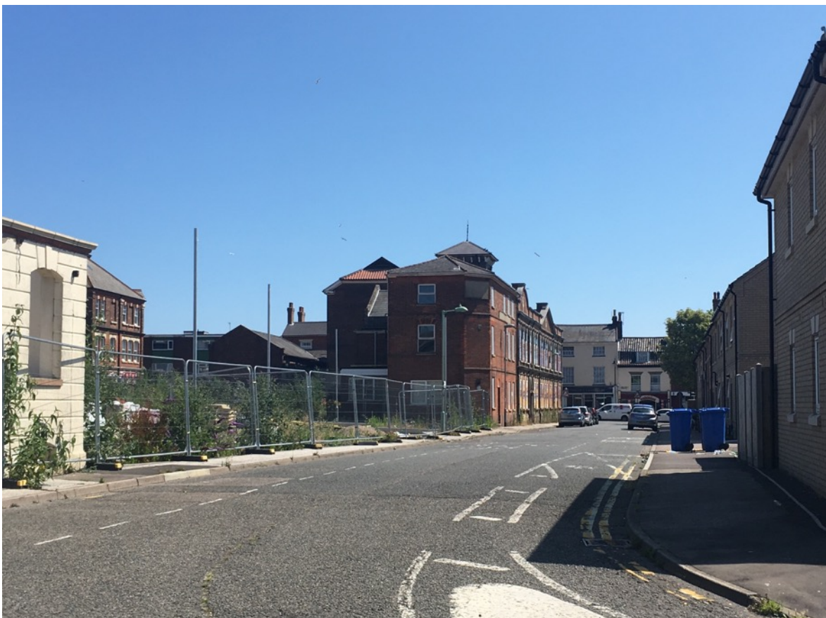
Figure 10: Town Hall from Compass Street, 2 Compass Street to centre, Coopers warehouse to left
