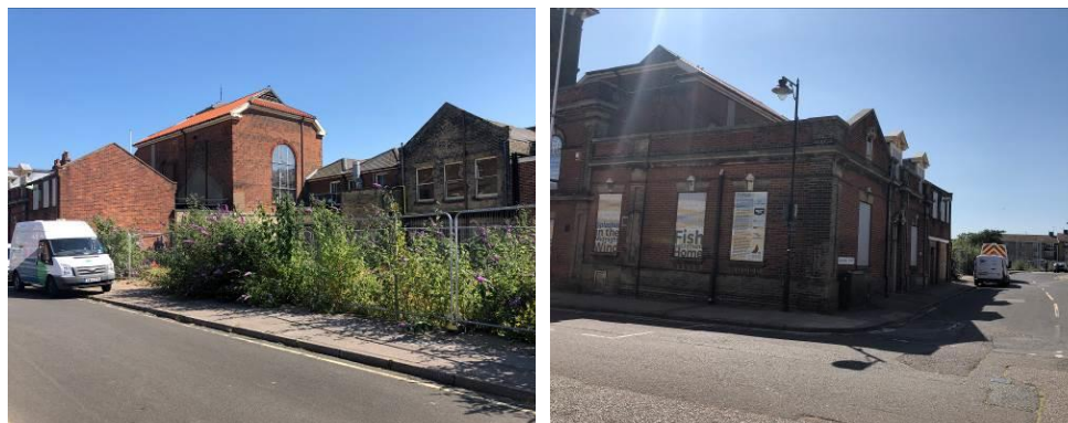
Figure 15: Mariners Street Extension
