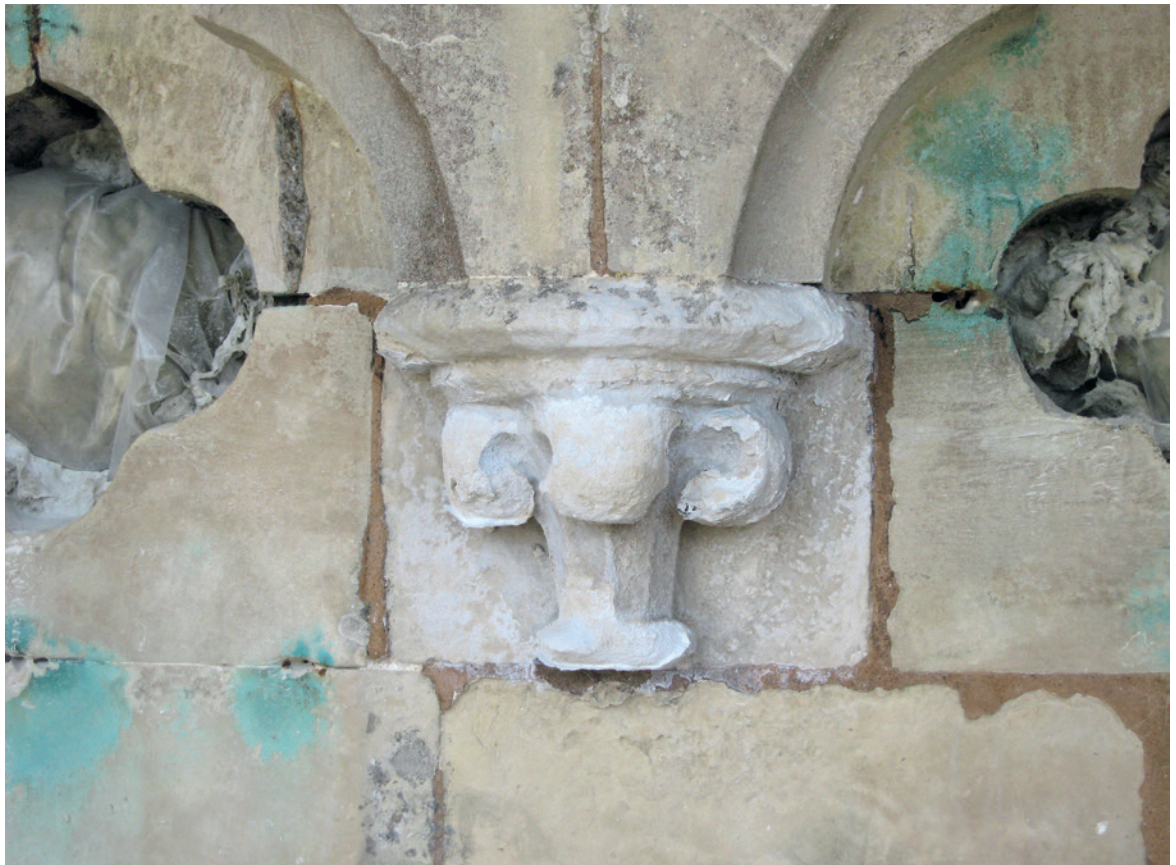
Nanolime has been used in of trials of consolidation of decayed Chilmark stone corbel at Salisbury Cathedral.
