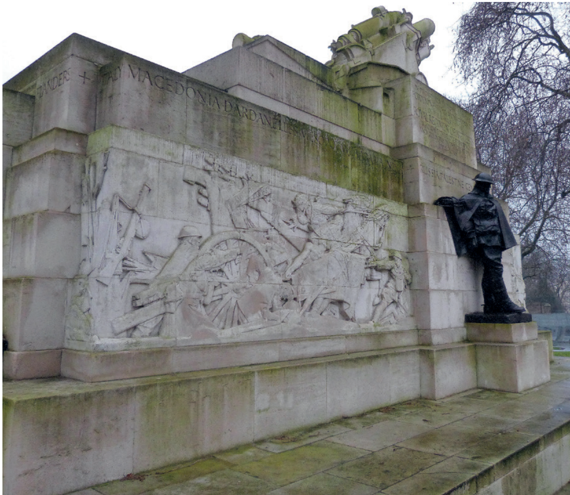
The Royal Artillery war memorial in London's Hyde Park, showing the carved area treated with Brethane being free of algae
