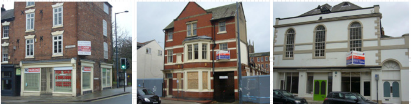
Empty units in historic buildings: Bold Lane / Cheapside 2010
