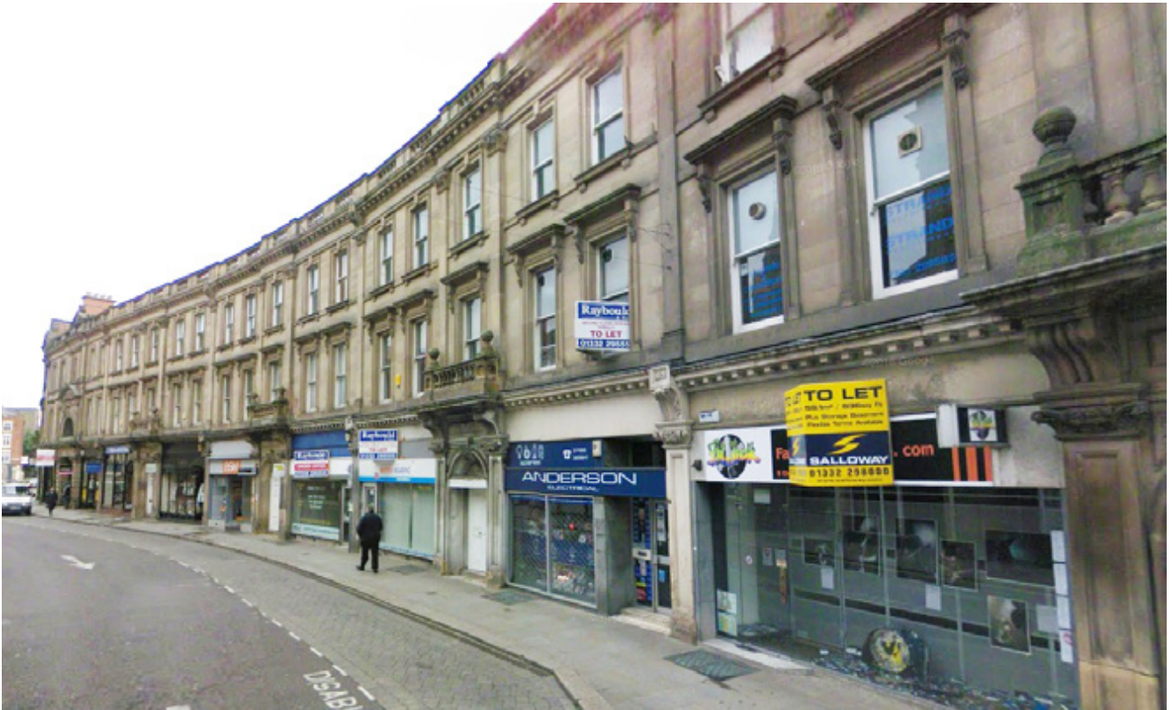
10 - 28 The Strand, Derby prior to multiple shop front repairs and reinstatement
