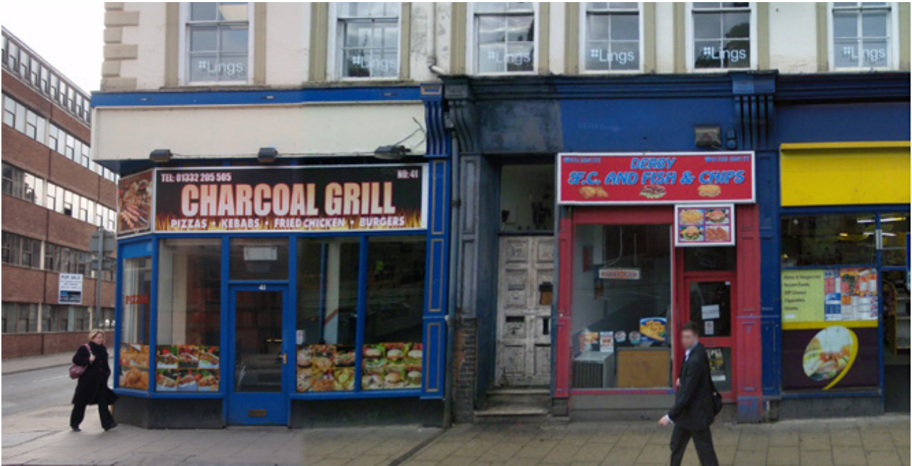
41-47 Wardwick, Derby before the shop front reinstatement
