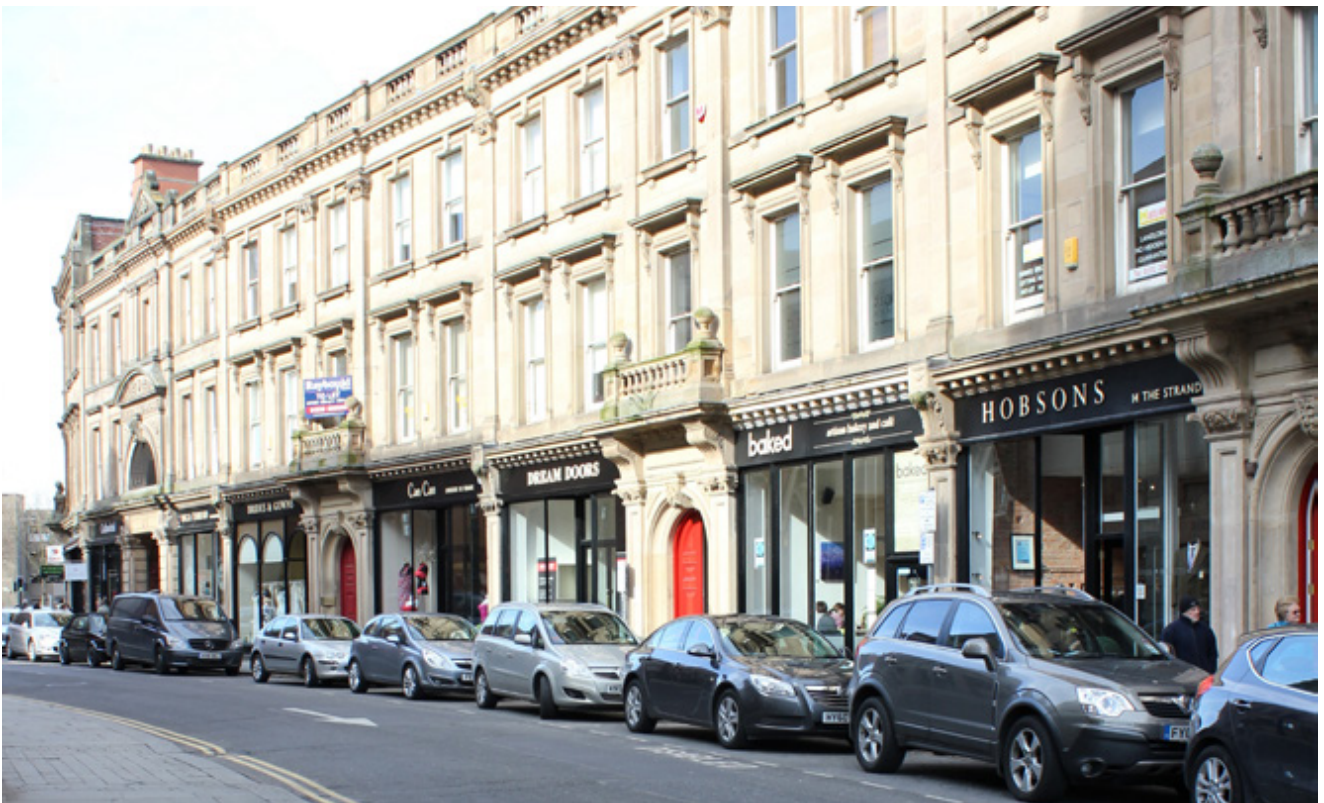
10 - 28 The Strand, Derby following multiple shop front repairs and reinstatement
