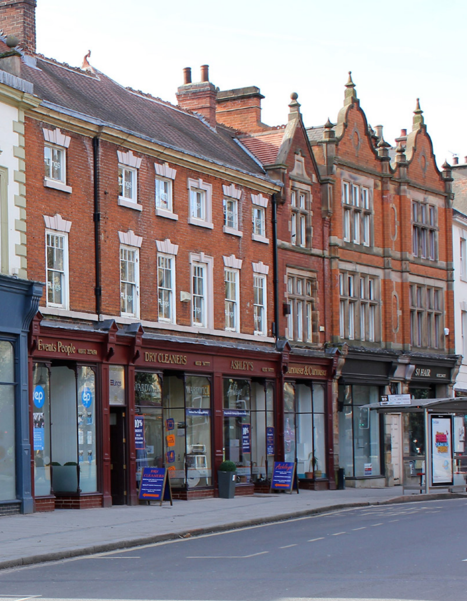
The newly reinstated shopfronts, 49-61 Wardwick, Derby
