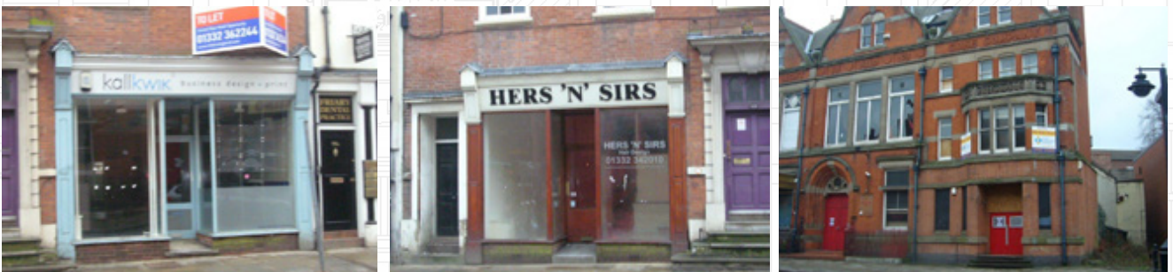
Empty units in historic buildings: Friar Gate 2010
