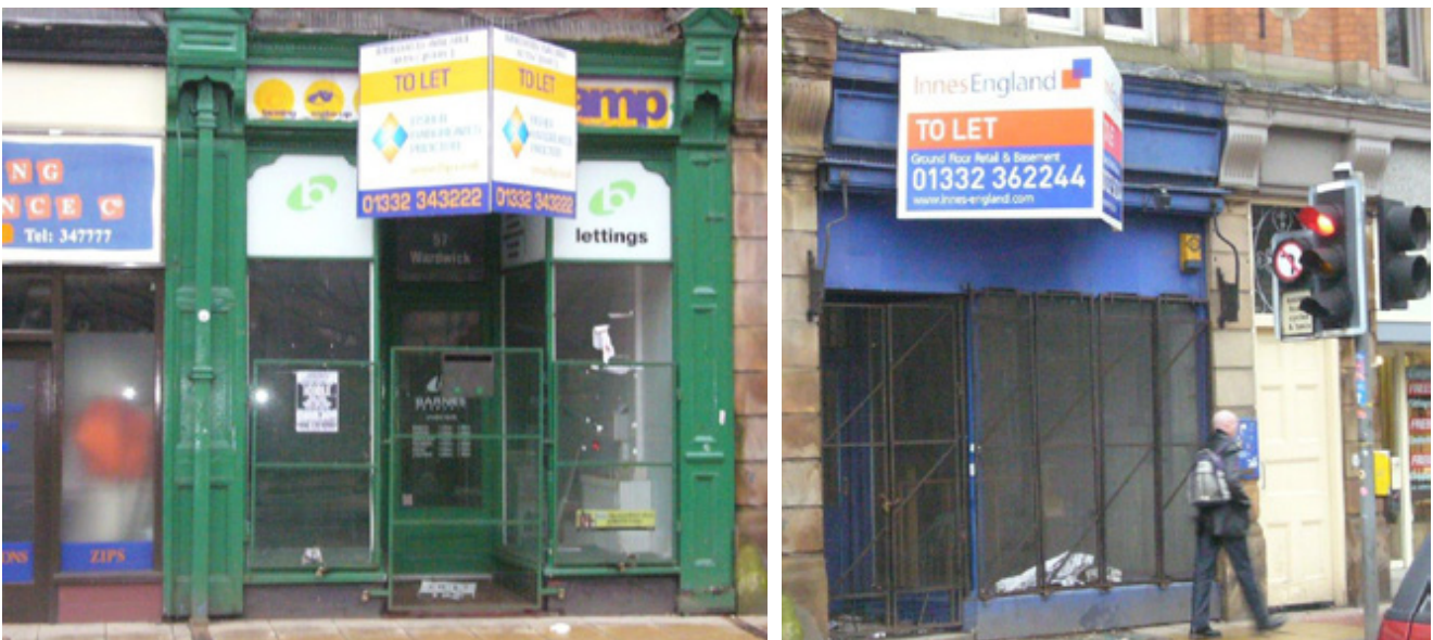
Empty units and inappropriate signage, Wardwick, Derby
