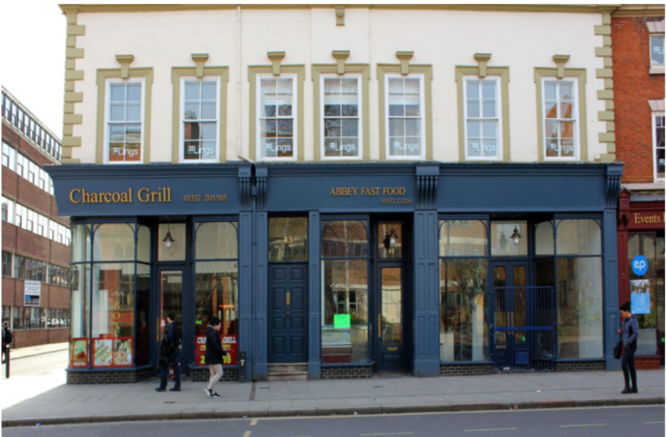
The newly reinstated shop front, 41-47 Wardwick, Derby
