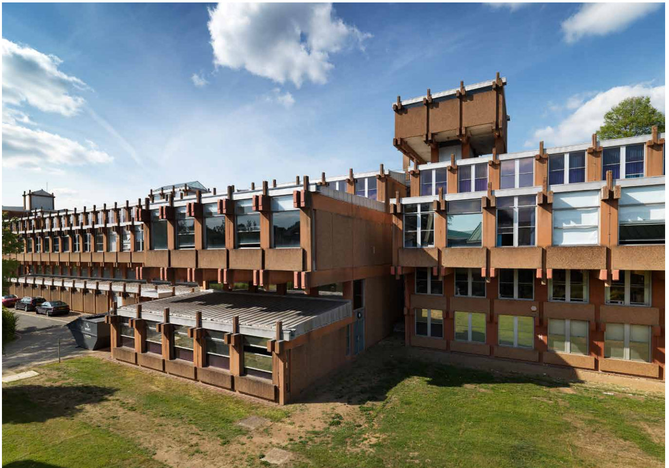
URS Building, University of Reading, 1970-72. © Historic England
