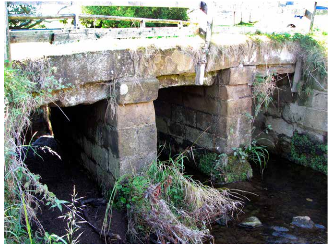
Clapper bridge, North Yorkshire, rebuilt 18th century. © Historic England
