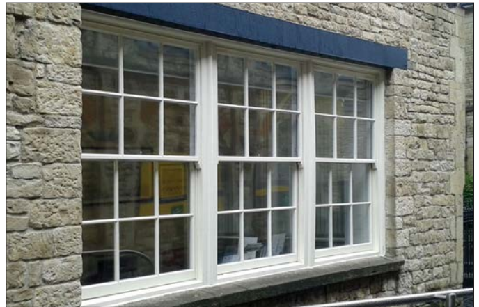
Timber sash windows, The Engine House, Swindon
