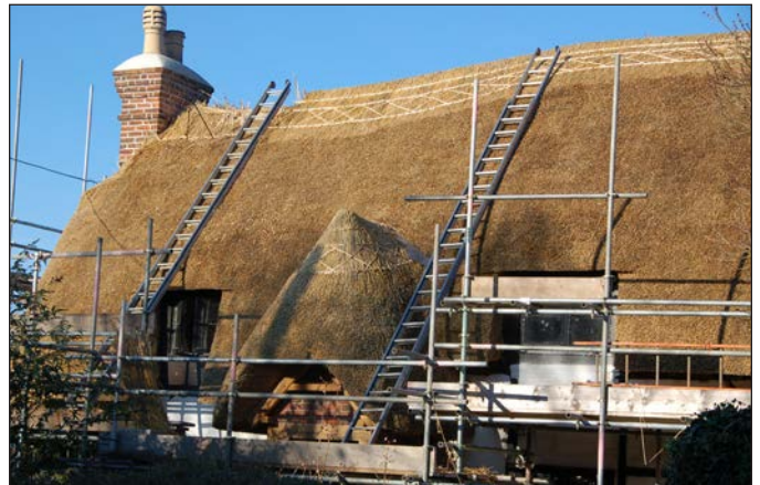
Re-thatching a cottage
