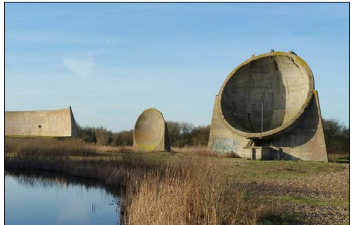
Concrete sound mirrors in Dungeness, Kent
