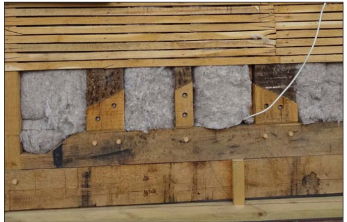
Insulation in timber-framed wall
