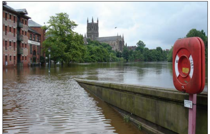
The River Sever overflowing its banks at Worcester
